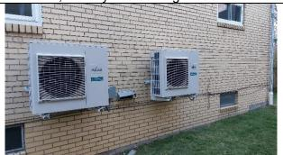
The old gas fired boilers that were used to heat the apartments have been removed. There was no cooling in the apartments. New energy efficient heating and cooling units have been installed for each apartment.
