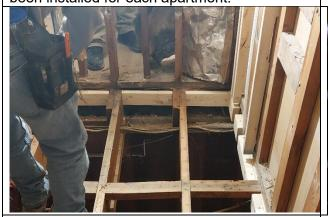
Where inspection revealed the need, floor joists and subflooring are being removed and replaced throughout all three buildings.
