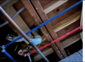
Both supply and drainage plumbing are being replaced and upgraded throughout all three buildings.
