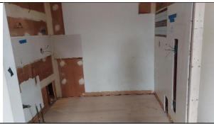
As part of the kitchen remodel the soffits, chimneys, and sections of wall were removed to allow additional cabinets, a dishwasher, and induction stovetop ranges to be installed.
