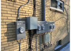
The electrical services for all three buildings have been upgraded. This includes meters, panel boxes, and the addition of new electrical circuits.
